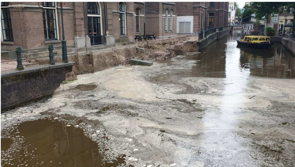
Figure 1.2: Collapsed quay wall at the Grimburgwal (Amsterdam) on September 1st 2020 (RTLNieuws, 2020).
