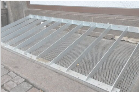
Slanting bars over heating vent
