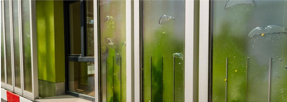
Figure 3: Solarleaf bioreactor facade (Wurm, 2012)
