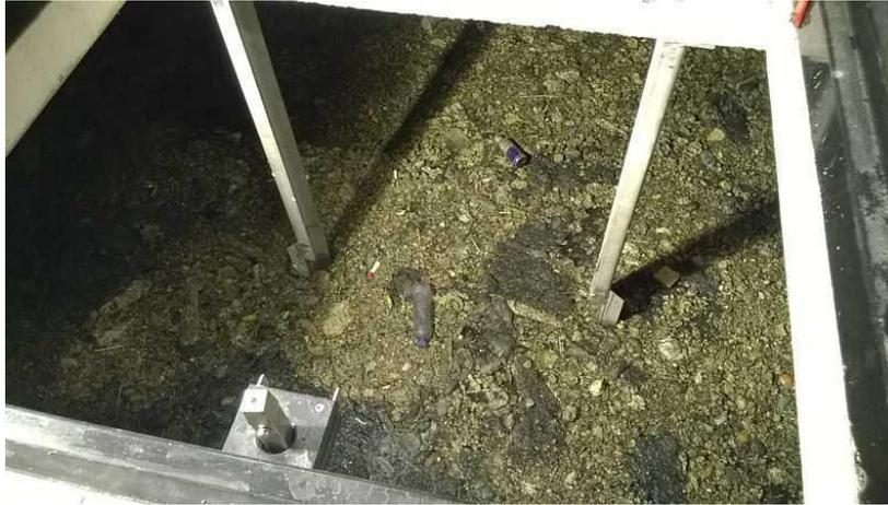
**Figure 1** The presence of a closed floating layer of scum and fat in a wastewater pump sump (Rotterdam, 2014)
