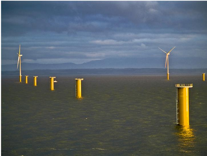
**Figure 1.5:** The construction of an offshore wind farm; the towers are placed on top of the transition pieces, they are connected at the platform at interface level.
