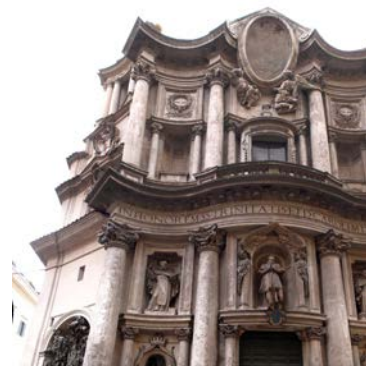
all drawings in scale 1:100 65. section of San Carlino 66. light section 67. floor plan of San Carlino 68. light plan 69. front facade of the San Carlino
