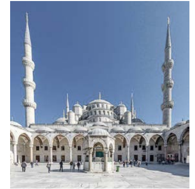
all drawings in scale 1:1000 70. forecourt of the sultan ahmed mosque in istanbul 71. light section 72. section of the sultan ahmed mosque
