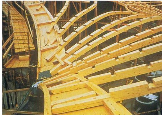
Figure 2.38: Box section under construction (Müller 2000)
