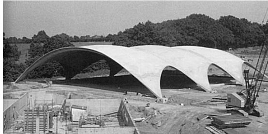
Figure 1.2: Shell structure by Heinz Isler<sup>3</sup>
