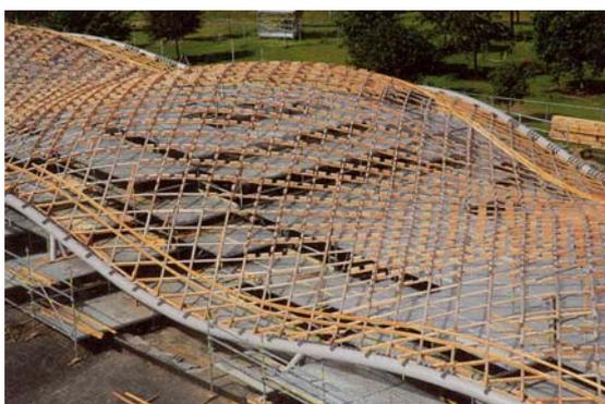
Figure 3.48: gridshell under construction (De Groot, 2007)
