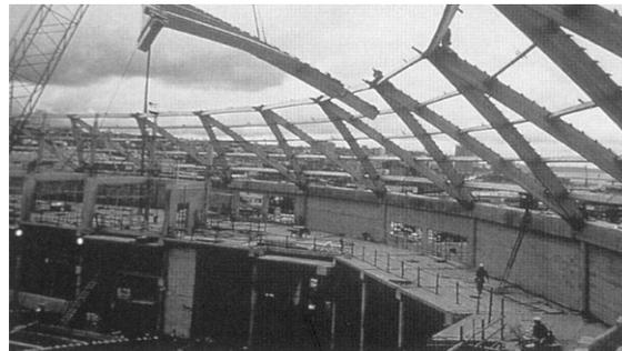
Figure 2.31: Tacoma dome under construction (Müller 2000)
