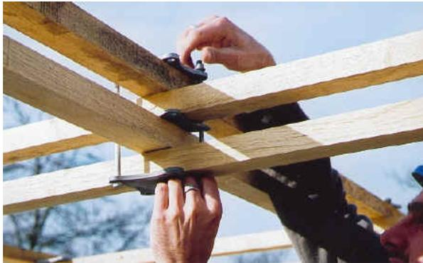
Figure 3.33: Assembly of a typical node joint<sup>14</sup>
