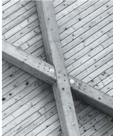
Figure 2.22: Node of the barrel vault lattice (Müller 2000)
