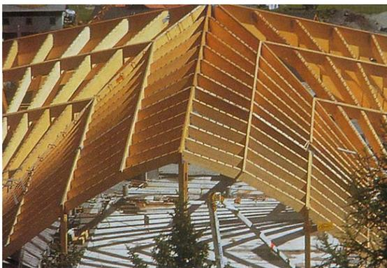
Figure 2.25: Davos ice rink under construction (Müller 2000)
