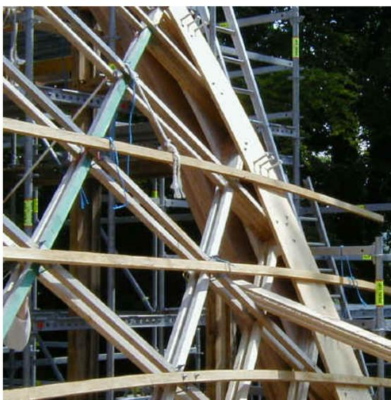
Figure 3.36: Connection to the edge<sup>14</sup>
