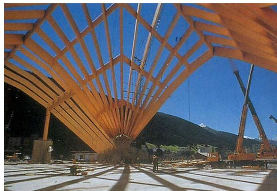
Figure 2.26 Davos ice rink under construction (Müller 2000)
