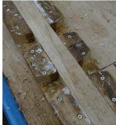
Figure 3.32: Scarf joint<sup>14</sup>
