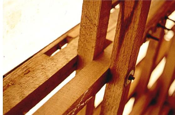
Figure 3.19: Photo of a typical node joint<sup>13</sup>
