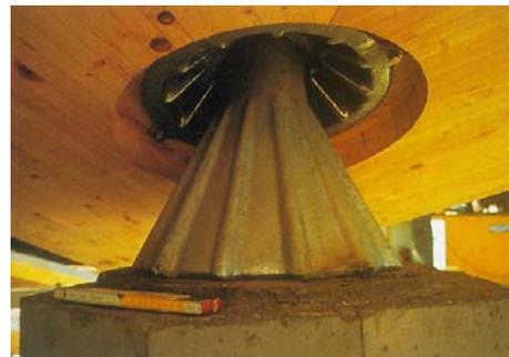
Figure 2.41: Cast steel bearing (Müller 2000)
