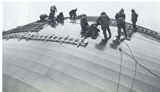
Figure 3.27: Applying the roof skin (Burkhardt et al 1978)
