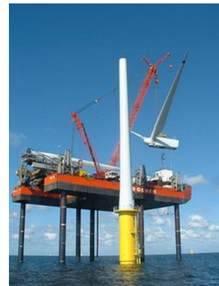
(f) Bunny ear assembly installation (Source- Seajacks)
