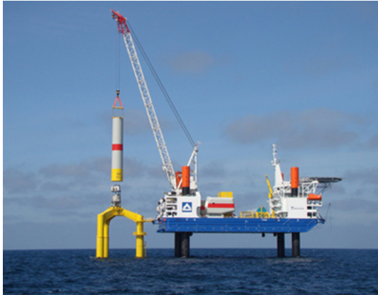
(a) Tower section installation (source-Offshore technology)
