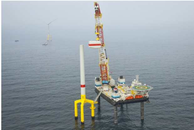
(c) Nacelle installation (source-Jack-up barge)
