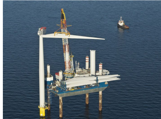
(b) Single blade installation (source-EDF Energy)
