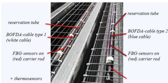
Figure 3. Instrumentation of the pile in formwork
