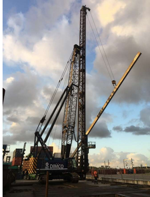
Figure 9. Pile before installation showing the slenderness of the pile
