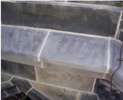
FIG. 2.14 Artificially patinated Bentheim sandstone on the lantern of the Laurens Church tower in Rotterdam / Photo: T.G. Nijland
