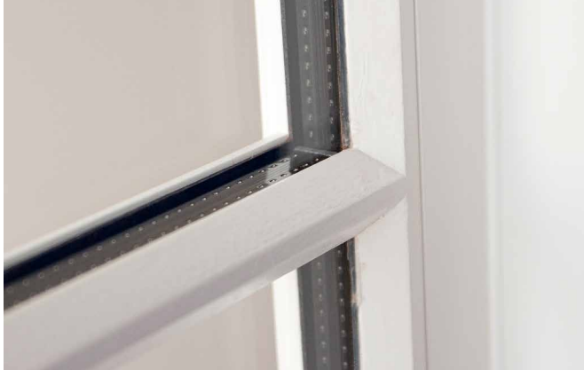
FIG. 5.33 Attached glazing bars are used when the existing structural bars are not wide or deep enough to accommodate double glazing
