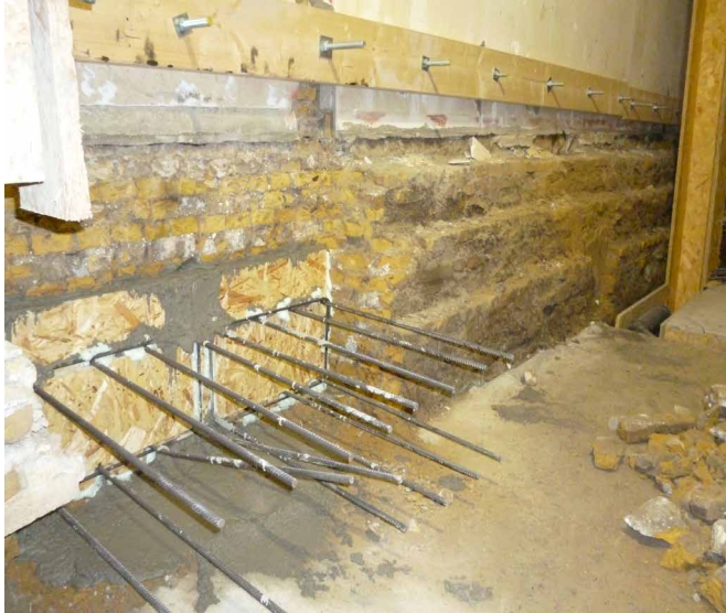
FIG. 3.10 Huis Nolet, basement: reinforcement for insertion of concrete floor (December 2016) / Photo: B. L.ubelli
