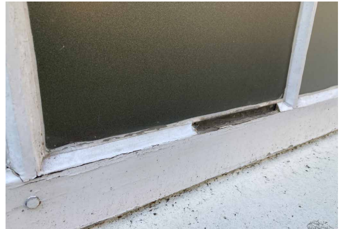
FIG. 5.18 Puttyed glass in wooden windowframe (in need of repair) / Photo: W. J. Quist
