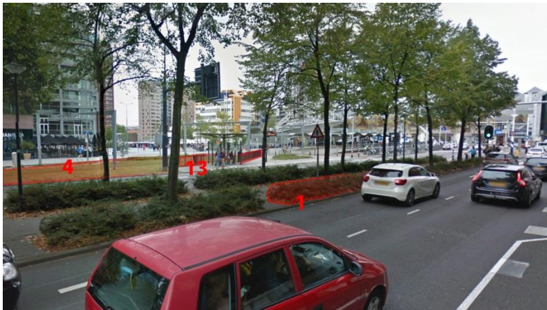
Figure 15 Example of uses and arrangement of elements (own ill.). Right to left: raised green separation, protective fence and separating grass.
