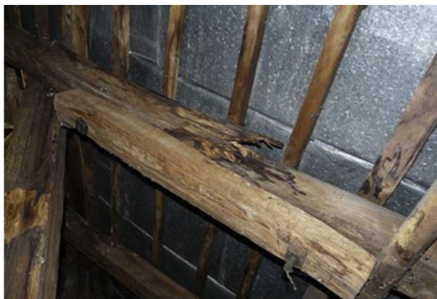
Image 6: Rotten wooden rafters (Mosoarca & Gioncu, 2013).
