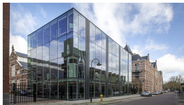
Image 15: Building D(emountable); building designed to be disassembled (cepezed, 2019)
