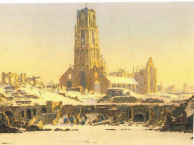
Demolished Sint-Laurens Church. Source: Historische Atlas van Rotterdam
