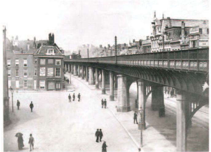
Elevated train track. Source: Historische Atlas van Rotterdam
