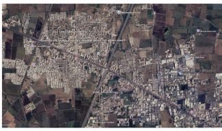
Railway through settlement areas
