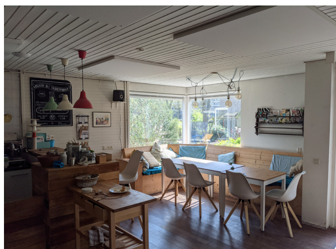
Figure 22: Acoustic ceiling panels compensate for the changed functionality of the room
