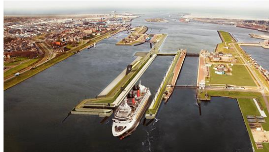
Figure 32 New Sealocks at IJmuiden (Dyckerhoff Basal, n.d.)
