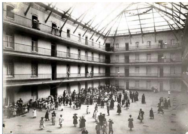
Figure 2b: Internal courtyard at the familistère (1863)
