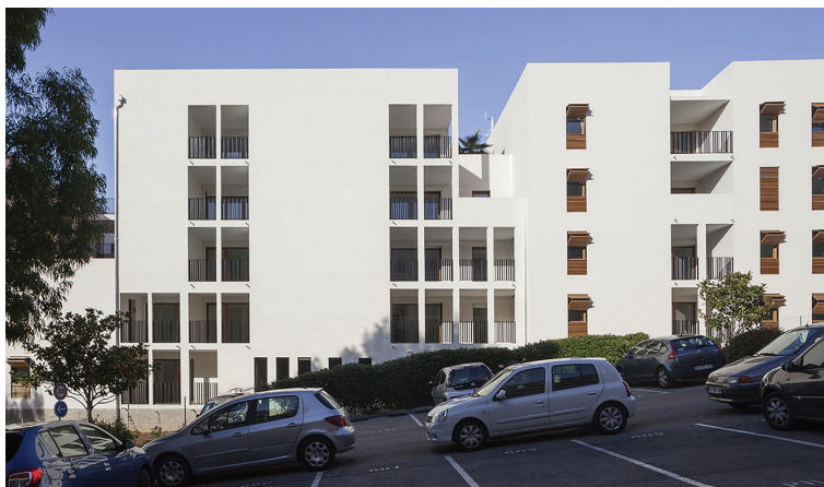
2) 58 Social Housing in Antibes / Atelier PIROLLET architectes
