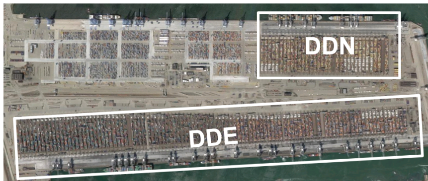
Figure 1.3: Layout of the Delta Terminal with northern side, DDN, and southern side, DDE
