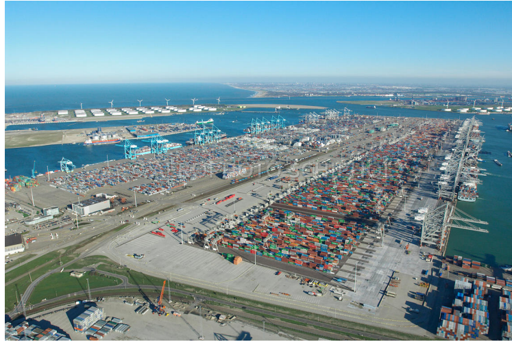
Figure 1.1: ECT Delta Terminal with quay cranes (right side), automated stacking cranes (left side) and AGVs (in between)
