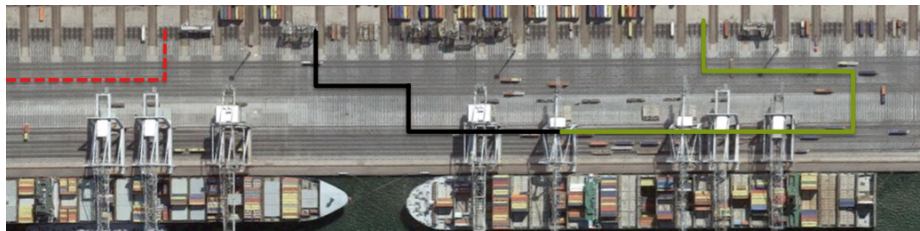
Figure 1: AGV movements during a discharge trip in black and green and during tanking in red
