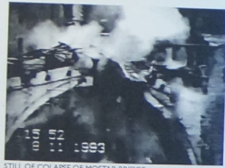
STILL OF COLAPSE OF MOSTAR BRIDGE
