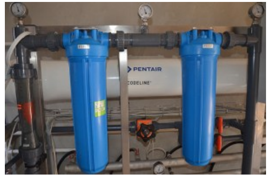
(b) [Pre-filtration] will prevent larger polluting particles to enter the RO, which is an easily clogged membrane. To avoid frequent membrane replacement, the pre-treatment will be designed for your site-specific situation. This can involve sand filtration, cartridge filtration, and more
