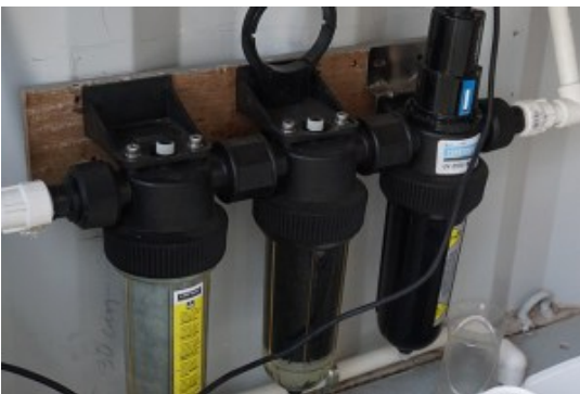
(e) [Post-treatment] is possible specific applications that can add fresh water treatment steps to the system, for example, remineralization, UV treatment before end use, or preservation dosing to make it suitable for longer-term storage.
