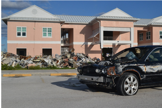
(a) Destroyed school building on the university campus that had been flooded by a storm surge credit; T. Özdemir
