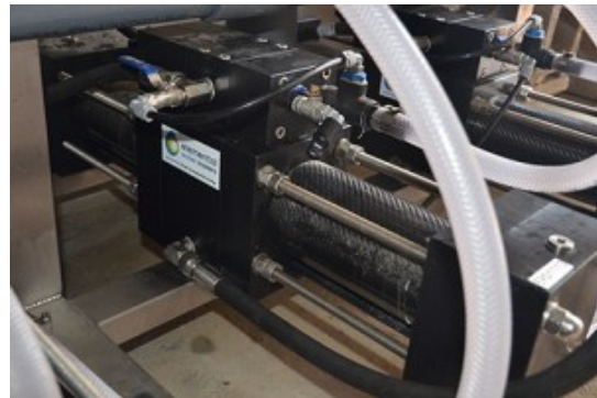
(d) [Energy recovery] enables re-using of the brine pressure. The already high pressure present in the runoff water makes it possible to reuse that same energy again. Energy recovery helps recover some of the energy typically lost from the pumps and membrane system. The primary objective is to recover much of the energy held in the pressurized RO concentrate stream. Before continuing to disposal or treatment, the concentrate is sent through an energy recovery device, and the recovered energy is used to partially power the pumps. [Greenlee et al., 2009]
