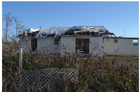
(d) Outside a destroyed residential house flooded by storm surge of Dorian credit; F. Ortiz
