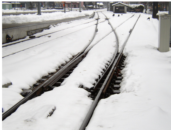
Figure 12: The switch rails can freeze to the stock rails if the heating is not functioning properly (Wikipedia, 2019)
