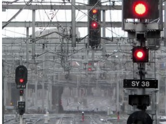
Figure 15: A signal failure will bring the signals to the most restrictive aspect (Freepik.com, 2018)
