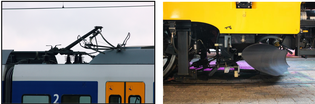
(a) A broken pantograph will lead to a serious disruption (Brouwer, 2013) (b) An object on the tracks could damage the ATP receiver (Sweekhorst, 2015)
