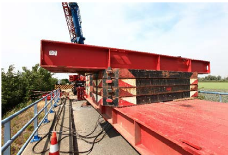
Figure 3. Proof load testing of viaduct Zijlweg [5]
