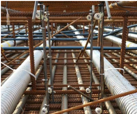
Figure 2. Smart aggregates in rebar cage.
