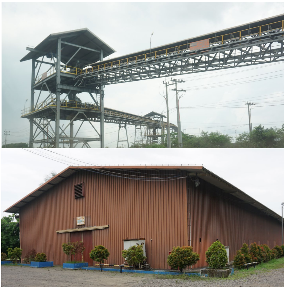
Conveyor system and Warehouse building.
