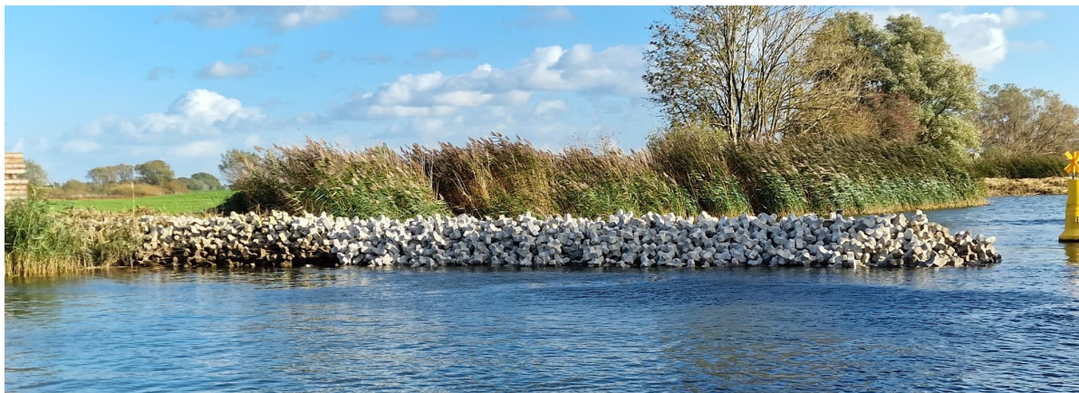
Figure 1.4: Extended flexible groyne in the river IJssel where the dark coloured Xstream elements on the left used to be the groyne before extension.
