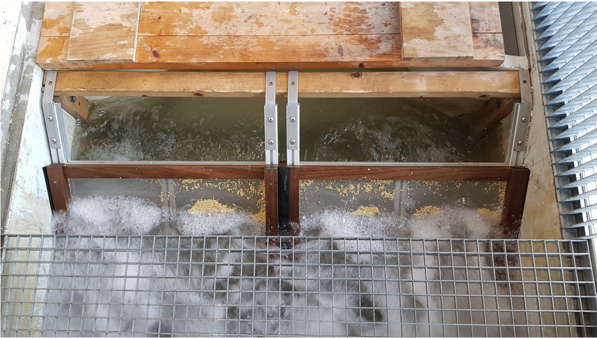
Filters to prevent suspended sediment ending up in the large reservoir
