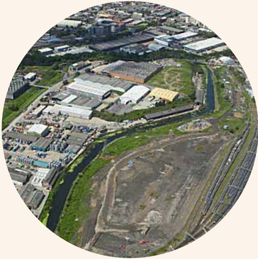
Stratford railway depot & industrial park
