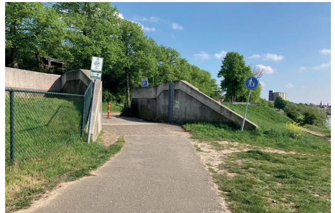
Image 11 - Quay walls in Venlo with slots for emergency walls
