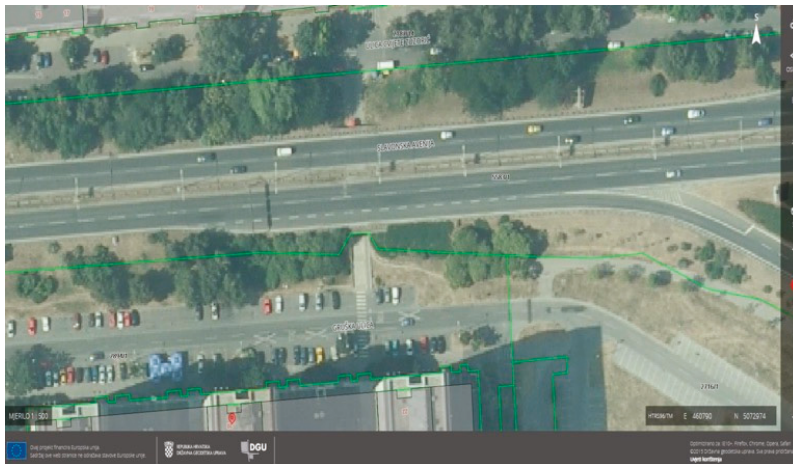
Figure 12. Pedestrian passage under the street in Zagreb, Savica, on the State Geodetic Administration Geoportal (digital orthophoto image overlapped with digital cadastral map) [37].
