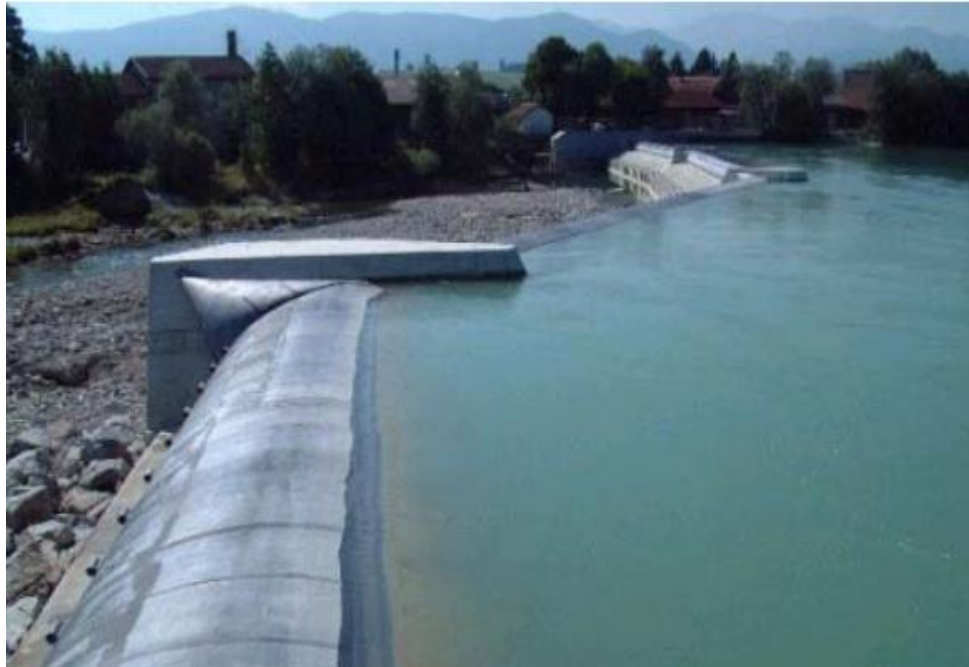
Figure 4-12: Rubber dam at river Lech, Germany [35]
