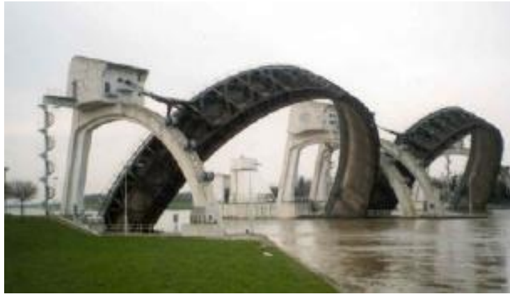
Figure 4-3: Rhine visor weirs, Hagestein, the Netherlands [28]
