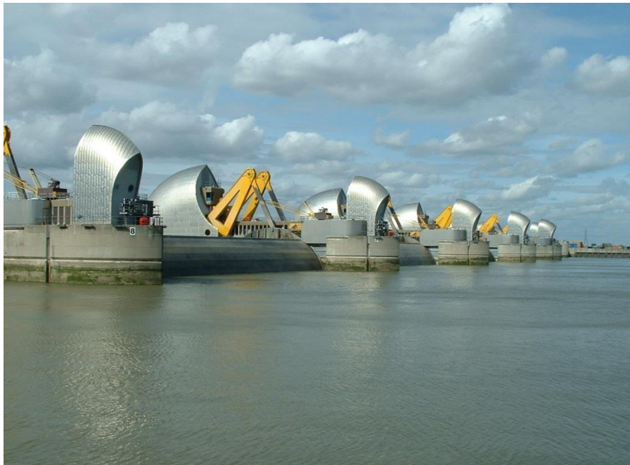
Figure 4-6: Thames barrier, London, UK
