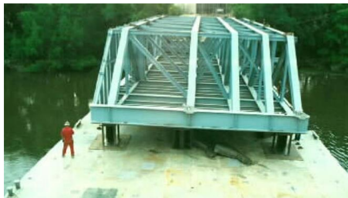
Figure 4-20: Bulkhead ready for shipment to the site [41]
