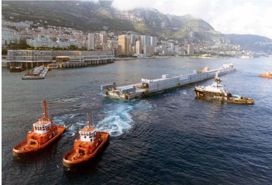
Figure 12-7: An example of the transportation of a caisson by using the tugboats
