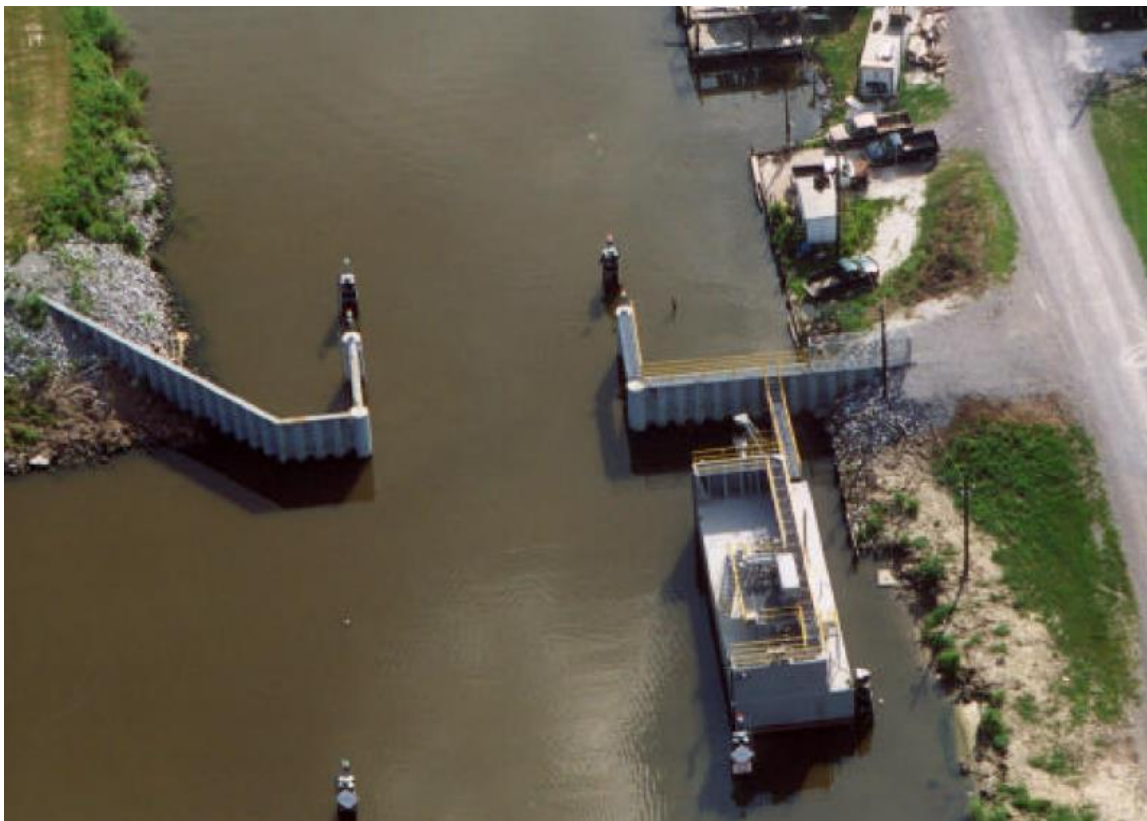
Figure 4-21: Bayou Dularge Barge Gate, Lockport, Louisiana, US [42]
