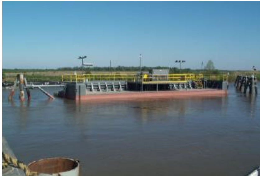
Figure 4-22: Bayou Lafourche Barge Gate in open position, Lockport, Louisiana, US [43]
