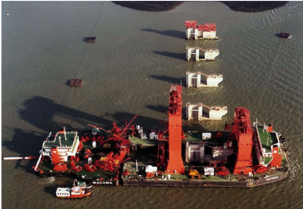
Figure 12-6: Placement of the piers in Easternscheldt barrier
