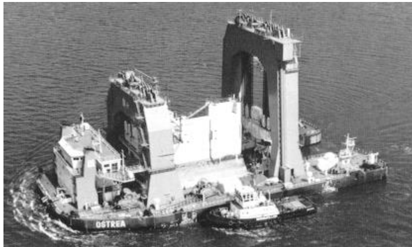
Figure 12-3: Floating crane Ostrea transporting a pier of the Easternscheldt barrier [80]
