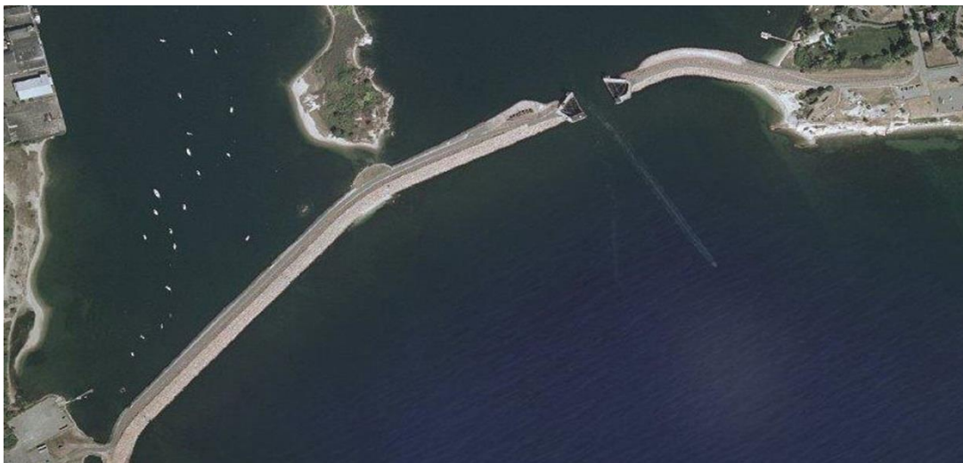
Figure 4-18: New Bedford Hurricane Barrier, Massachusetts, US
