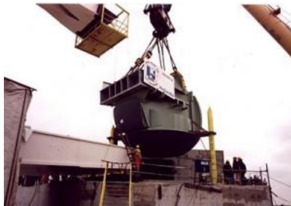
Figure 8-16: Maeslant barrier ball-joints articulation system [72]
