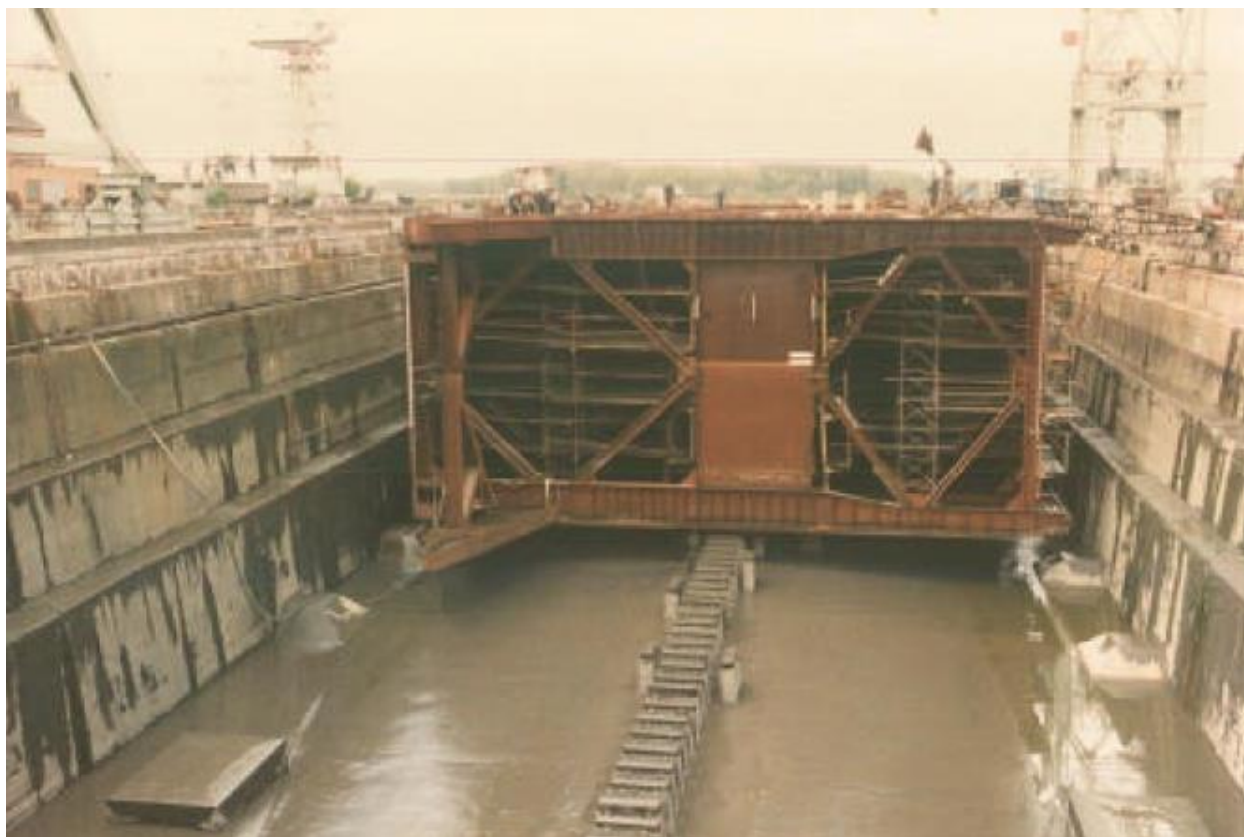
Figure 4-16: Lock doors during construction [38]
