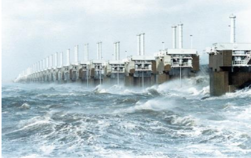
Figure 4-13: Eastern Scheldt (Oosterschelde) Storm Surge Barrier, the Netherlands
