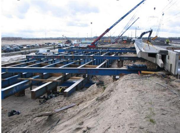
Figure 2-7 Horizontal jacking of a bridge deck
