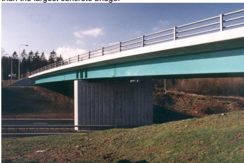
*Figure 3-3 Steel-concrete integral bridge*
