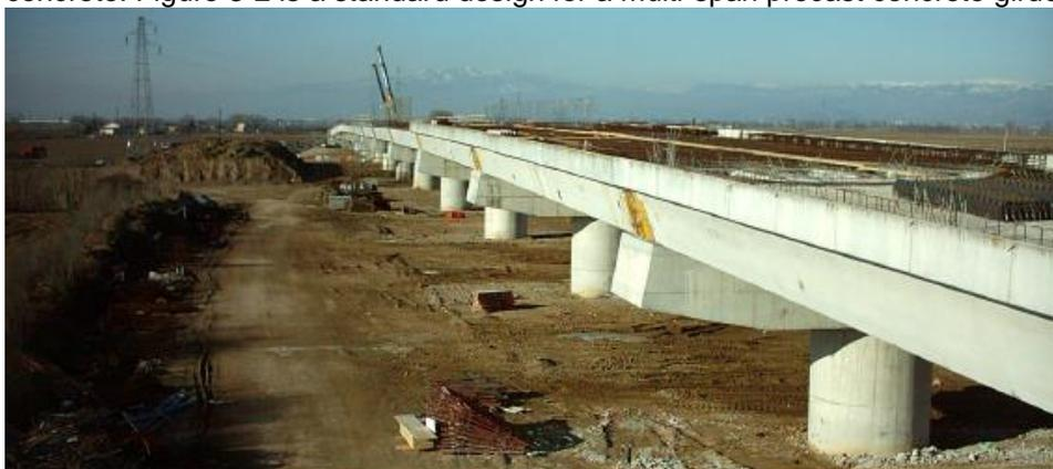
*Figure 3-2 Prefab prestressed concrete integral abutment bridge under construction*
