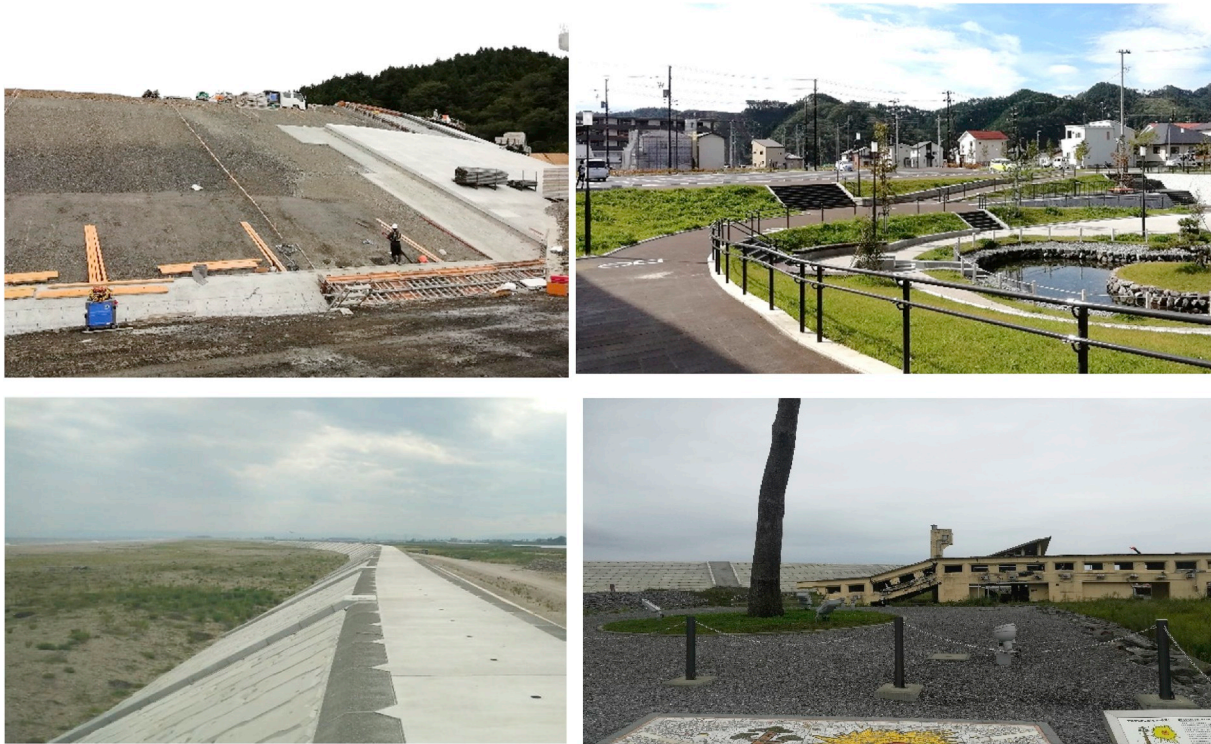
Fig. 2. Top left. Construction of new dyke in Otsuchi town (Sept 2018). Top right. New park in Otsuchi, showing the original level of the town (pond on the right) and the new level (houses at the back). Bottom left. Reconstructed dike along the Sendai plains coastline (photo courtesy of Glasbergen, T). Bottom right. New coastal dyke at Rikuzentakata, in front of a preserved memorial building.
