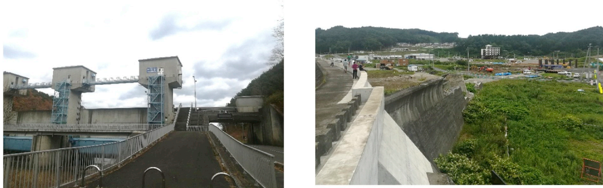
Fig. 1. Left: The dyke and floodgates at Fudai successfully stopped the tsunami, despite suffering some overtopping (inundation marks of \sim 20 m in front of the structure, indicated by the blue sign on the rightmost tower). Right: At Taro the massive coastal walls were overtopped, and the town behind them completely destroyed (pictures by authors). (For interpretation of the references to colour in this figure legend, the reader is referred to the Web version of this article.)
