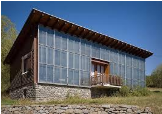
Fig. A.2. Jacques Michel's first Trombe wall house in Odeillo. François, M. (1967)
