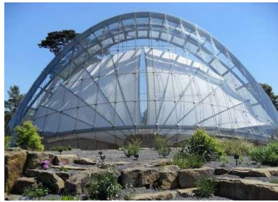
Fig A.10. Shading system of the Davies' Alpine House. Source: Environment - Davies' Alpine House (n.d.)
