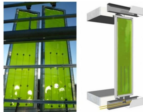
Fig. 11. Case model for algae façade in Hamburg, Germany. Source: International Building Exhibition
