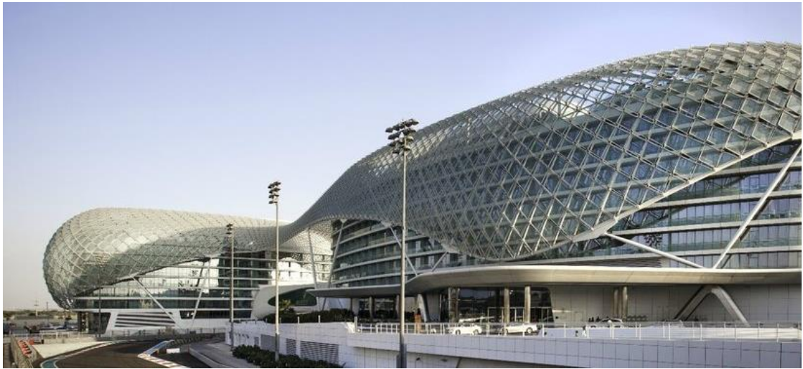
Figure 3: Example of a new building project: Yas Hotel (Abu Dhabi, UAE) © 2012 Waagner-Biro AG.
