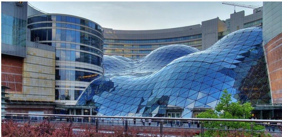
Figure 33: Exterior view of the undulating roof [34].
