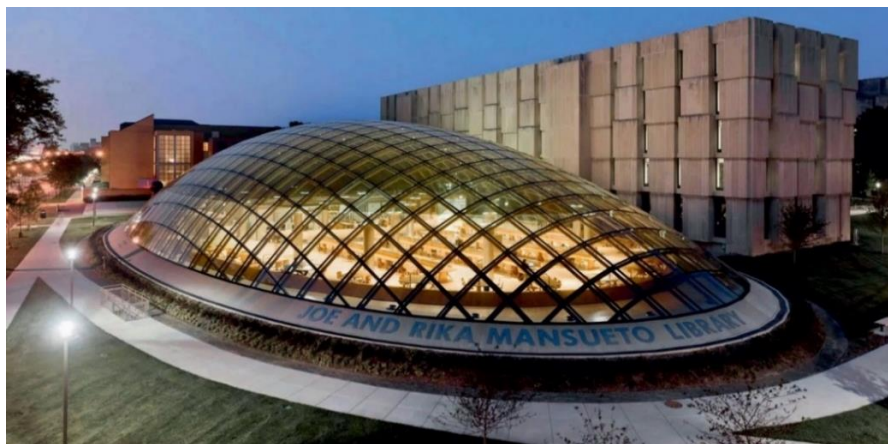
Figure 5: Example of a gridshell, Joe and Rika Mansueto Library, Chicago (2011) [6].
