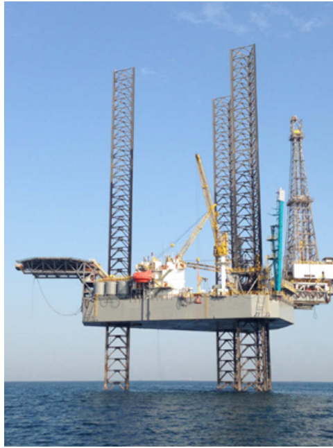
Figure 10: Jack-up elevated above the sea-surface (Offshore-energy, 2022)
