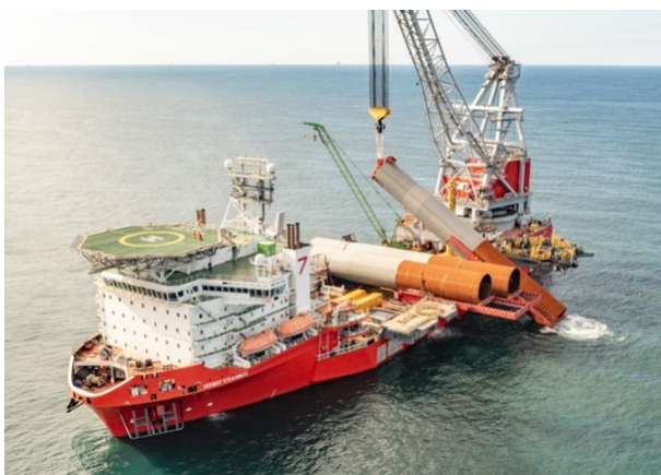
Figure 1: floating-vessel installing a monopile (Dogger-Bank, 2024)
