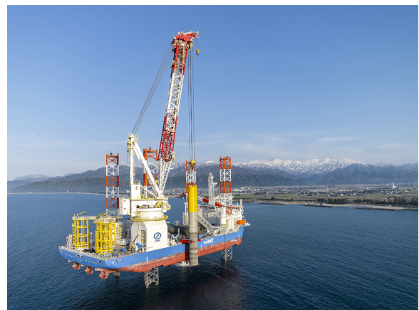
Figure 2: jack-up vessel installing a monopile (Wind-systems, 2023)
