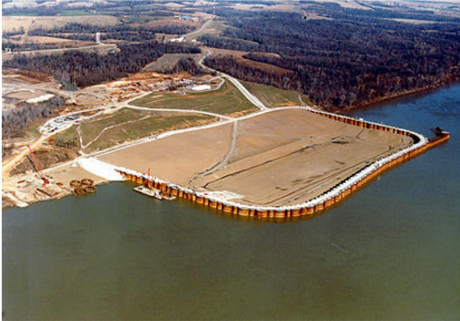
Figure I.3: Cellular sheet pile building pit for the construction of the Olmsted Locks and Dam
