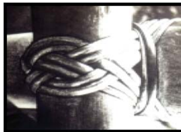
Joint with rattan lashing (Dunkelberg 1985)
