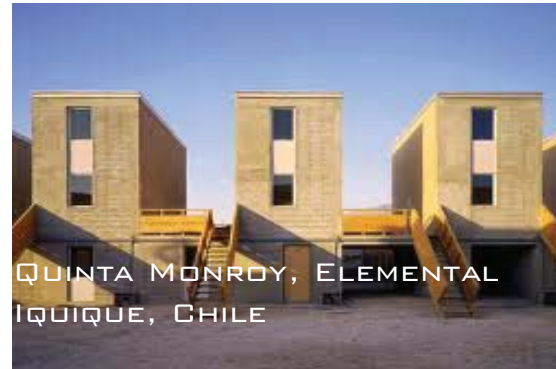
QUINTA MONROY, ELEMENTAL IQUIQUE, CHILE BUDGET: US $204 /SQM UNITS: 93 HOUSES SITE: 5000 M2 CONSTRUCTED AREA: 3500 M2
