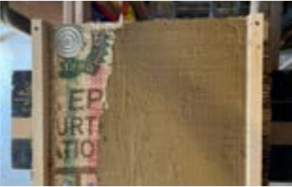
Finishing with clay plaster
