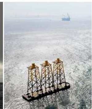
Figure C.3: Transport of Alpha Ventus jacket
