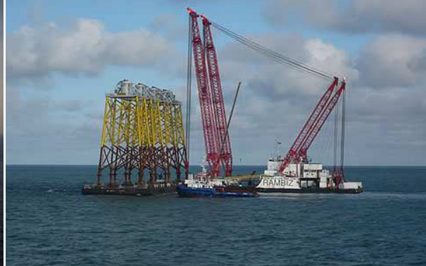
Figure 8.11: Transport of four jackets at Ormonde
