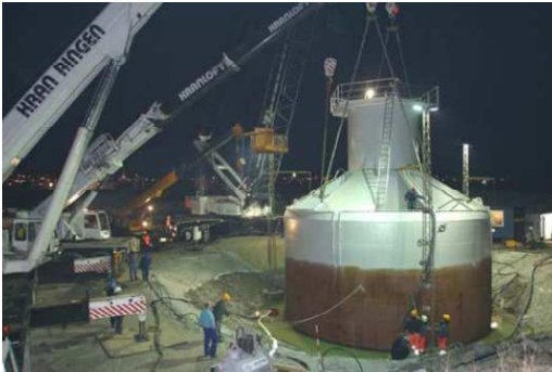
Figure 3.3: Suction bucket in Fredrikshavn
