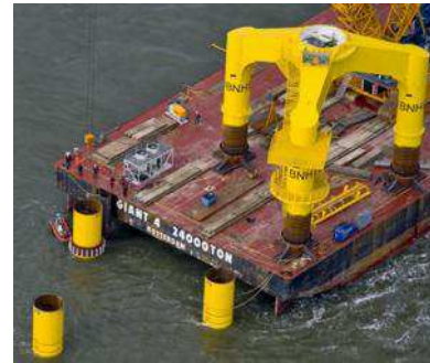
Figure C.7: Tripile installation
