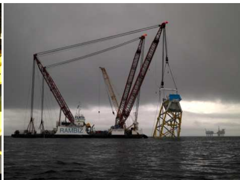
Figure C.2: Installing Beatrice Jacket
