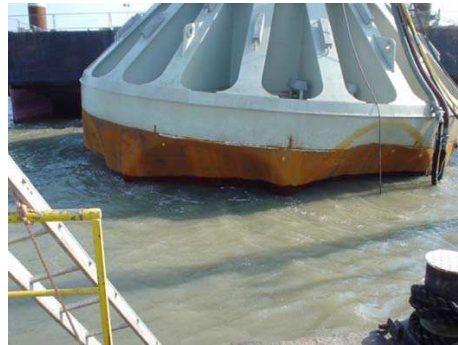
Figure B.2: Failed attempt during installation at Wilhelmshaven
