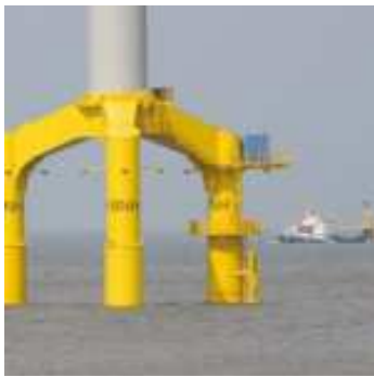
Figure C.6: BARD's tripile
