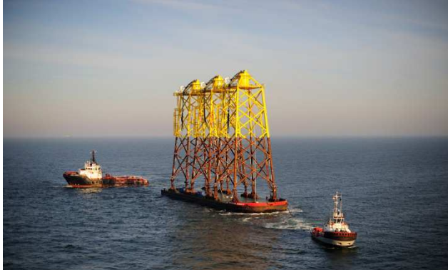
Figure 8.10: Transport of three jackets at Alpha Ventus
