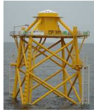
Figure 2.8: Transition piece Alpha Ventus
