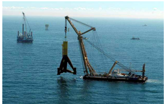
Figure C.5: Installation of tripod
