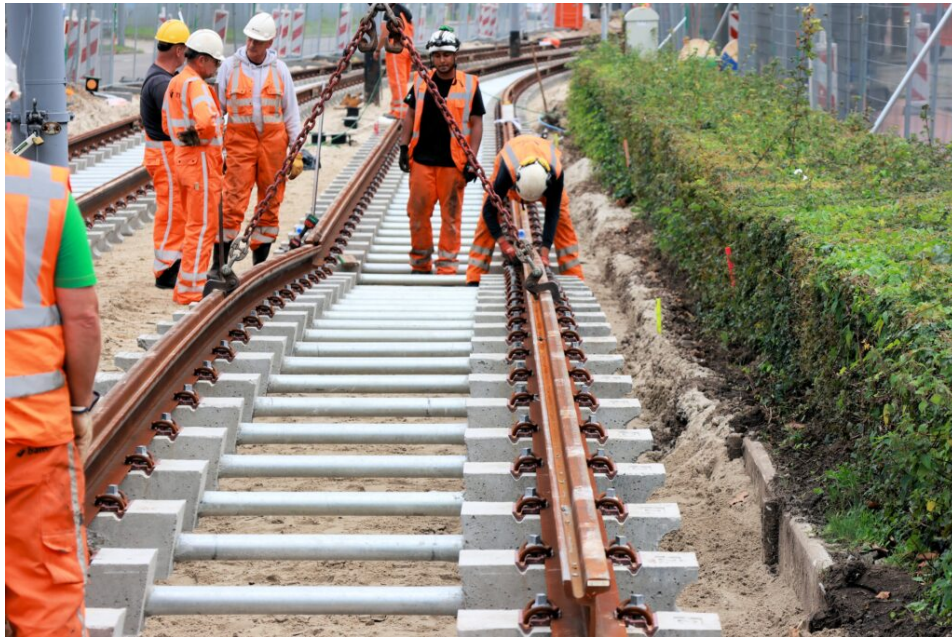
Figure 2.8: Placement of the duo-block sleepers and rails on the sand subgrade on the RET network [17]
