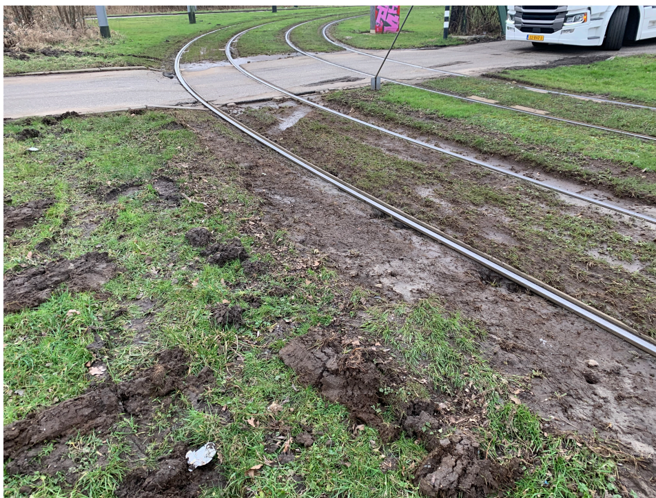
Figure 1.4: Settlements of the tram track in Beverwaard [2]
