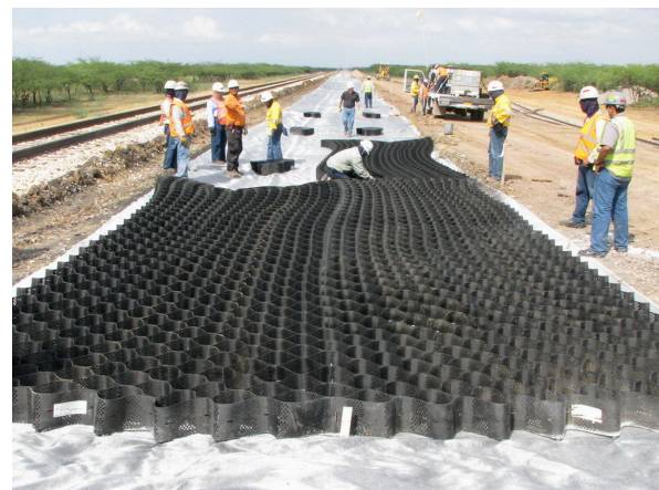
(b) Installation of geocells to stabilise the sub-ballast [66]
