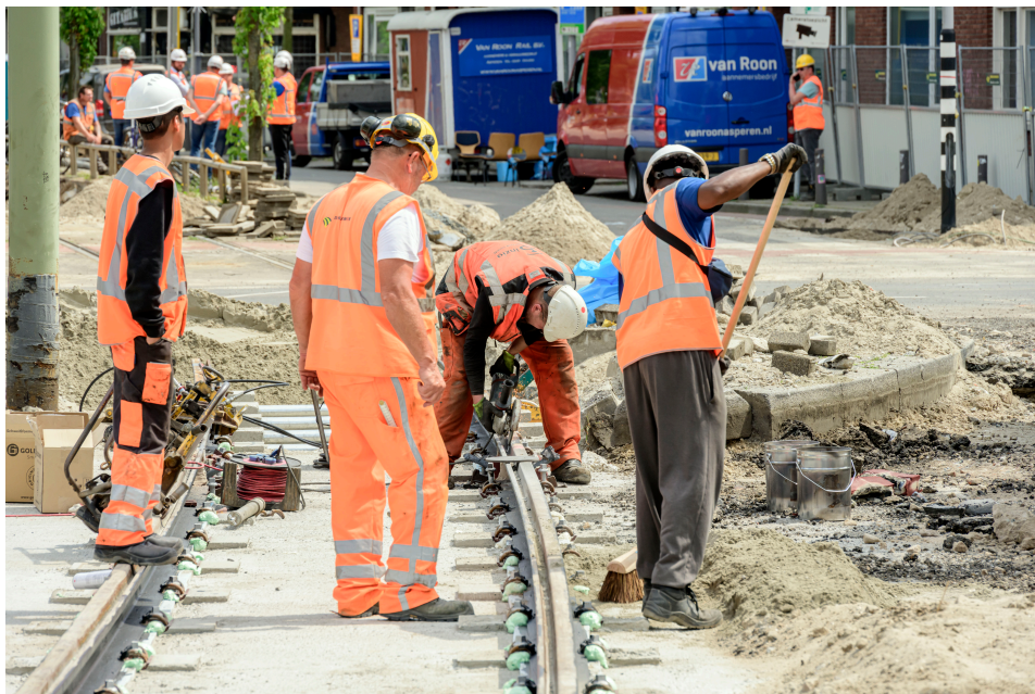
Figure 2.9: RET tram track structure after casting the concrete foundation plate [18]
