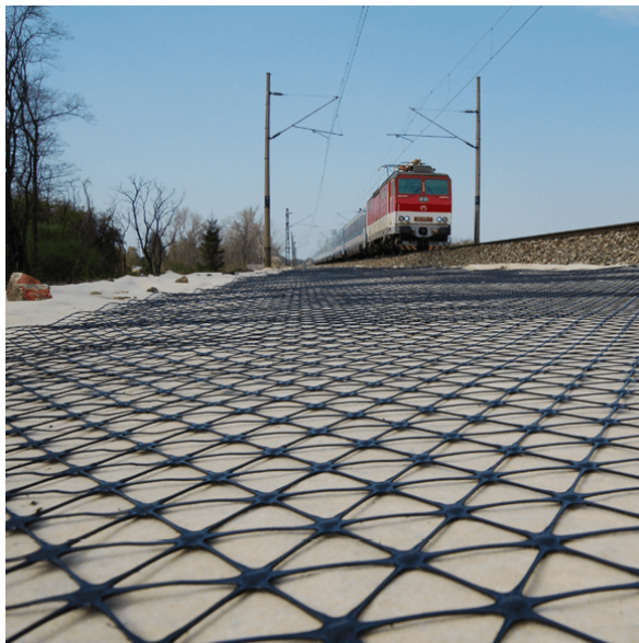
(a) Application of Tensar Geogrids in Romania [65]
