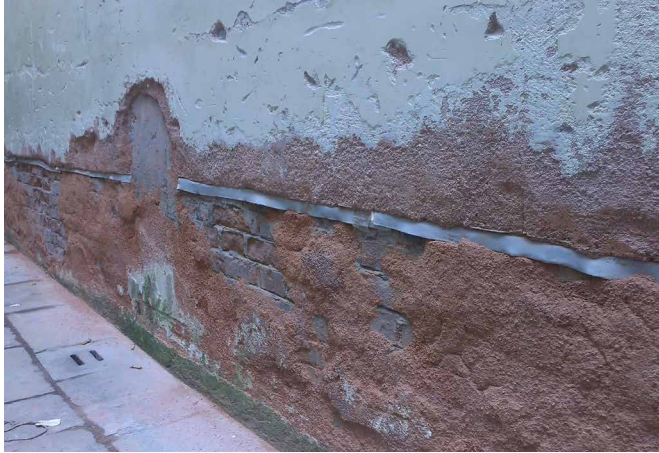
FIG. 3.3 Mechanical interruption of the wall by the use of plastic sheet, Venice, Italy / Photo: B. Lubelli
