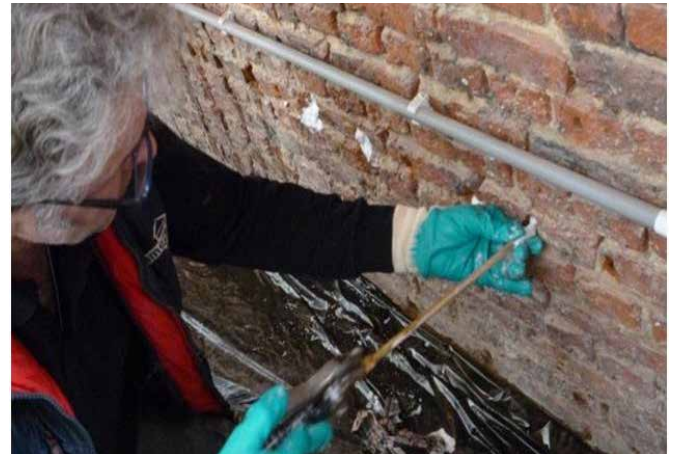
FIG. 3.6 Injection of a liquid product by means impregnation with a product in the form of a cream / Photo: B. Lubelli
