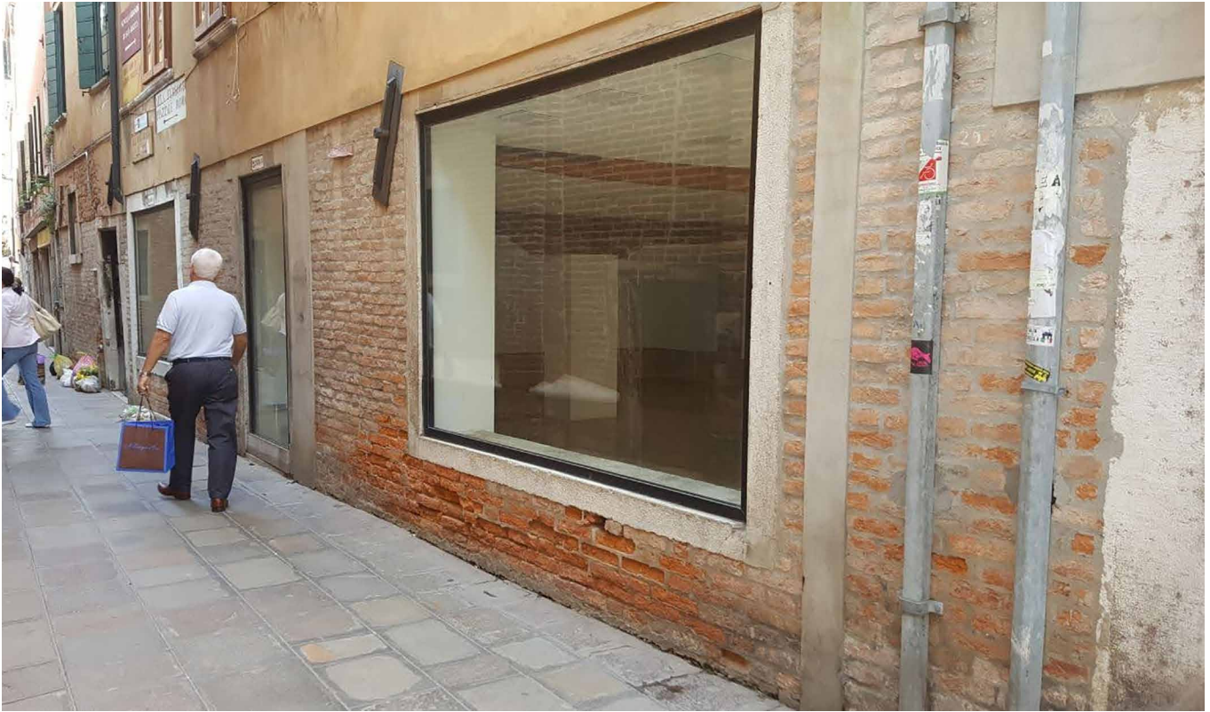
FIG. 3.1 Salt crystallization damage due to the presence of salts and rising damp, Venice, Italy / Photo: B. Lubelli
