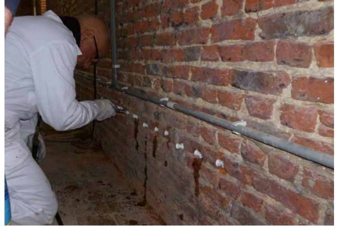
FIG. 3.5 Injection of a liquid product by means of pressure / Photo: B. Lubelli
