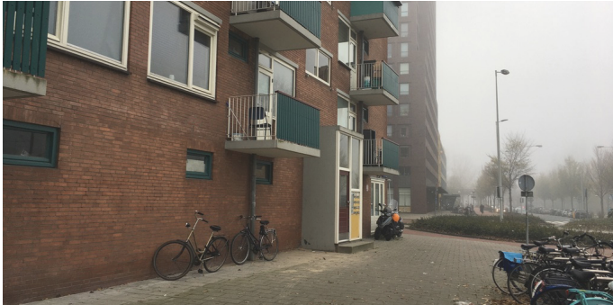
Fig. 53 Blind facades on the ground floor
