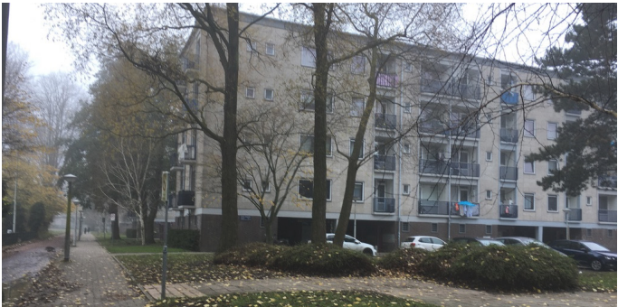
Fig. 58 Inaccessible green and blind facades on the ground floor
