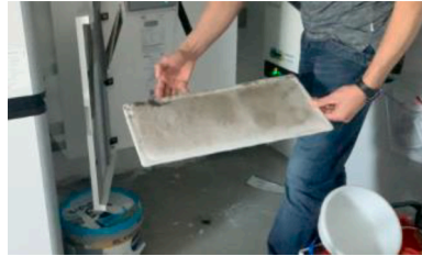
Fig. 7. Gideon shows the dust that settles on the air filters.
