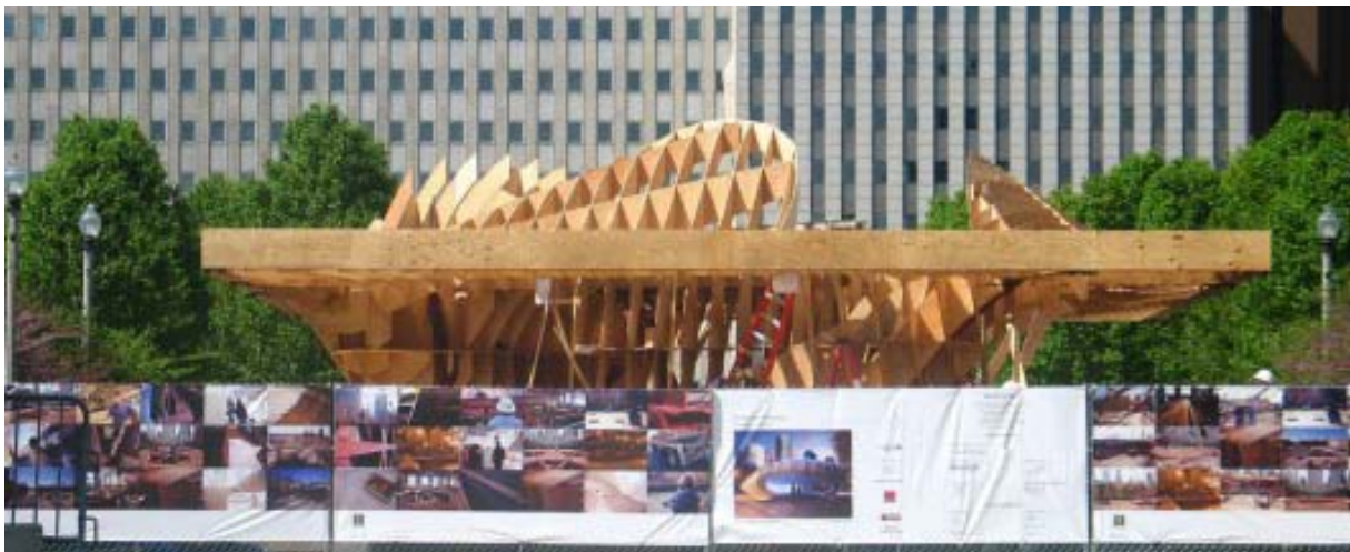
Figure 6: Building the Burnham pavilion designed by UN-studios
