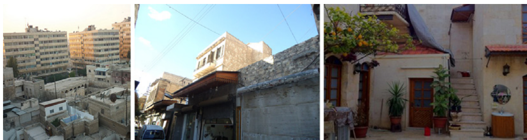
FIG. 3 Architectural anomalies and changes in functions made by inhabitants before the Syrian Civil War: adding rooms on the first floor, adding additional floors and changing the residential functions to commercial one, and adding a toilet and a bathroom in the courtyard (left to right). Source: author – field work 2010.
