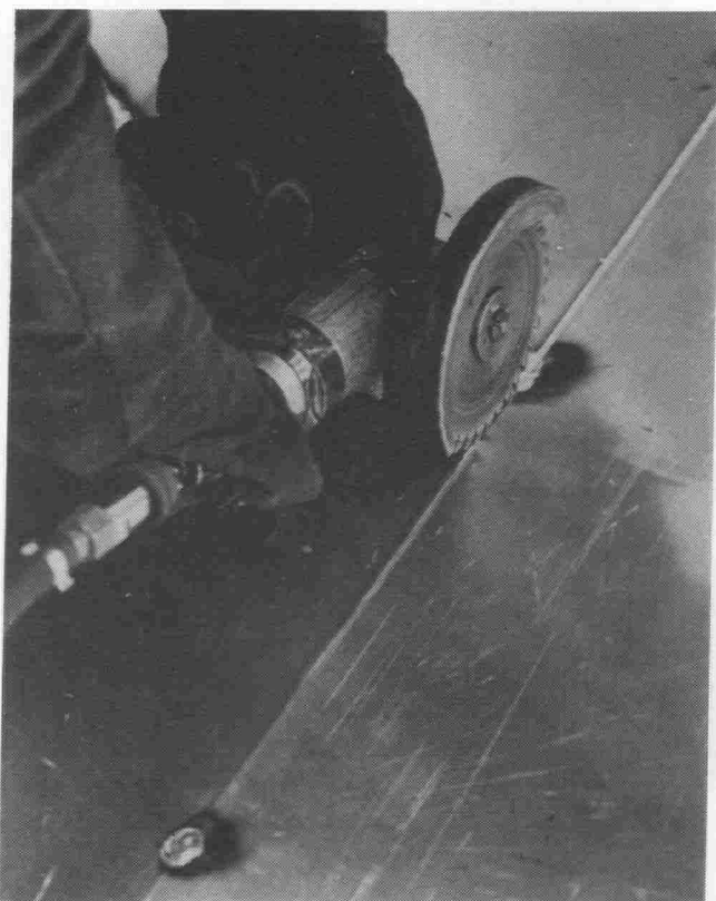
Photo 12. Cut-out the oppo site side with saw- equipment
