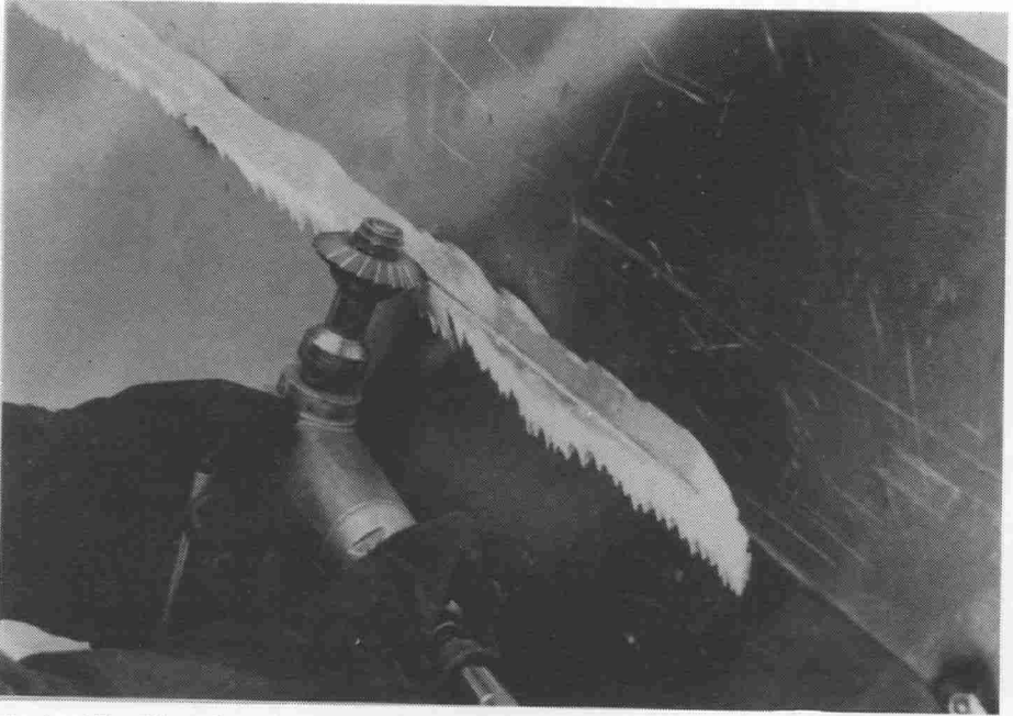
Photo 15. Cleaning the joint by brushing
