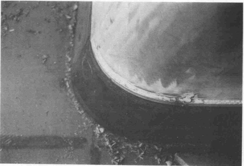
Photo 20. TRI-CLAD after bending and welding to aluminium and steel
