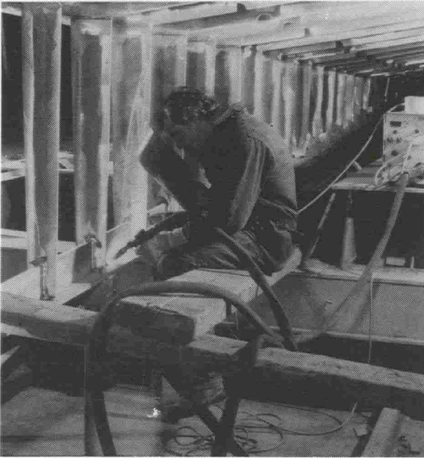
Photo 7. MIG welding with push-pull wire transport system
