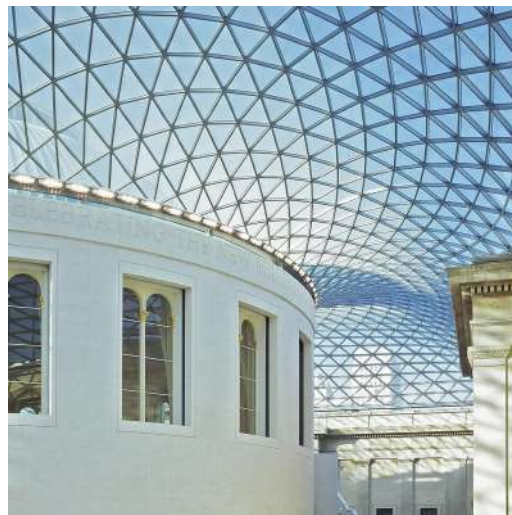
Figure 3.3: The triangulation of the Great Court Roof of the British Museum, via The Guardian
