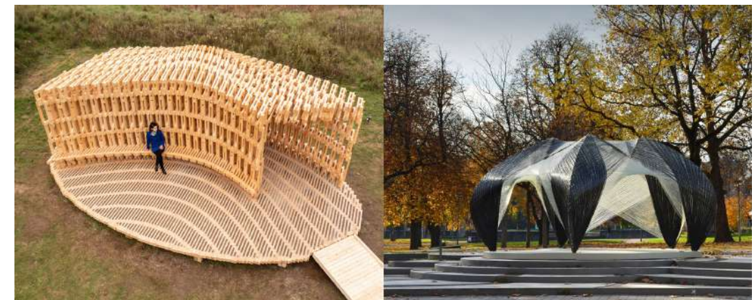
Figure 7.4: These pavilions are built using robotic construction processes, authors in text
