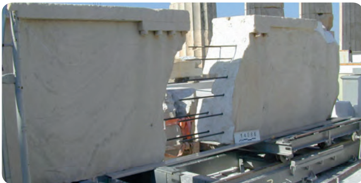
Figure 100: Reconstruction of a Frieze in the Parthenon, source: (Bouras, Ioannidou, & Jenkins, 2012)
