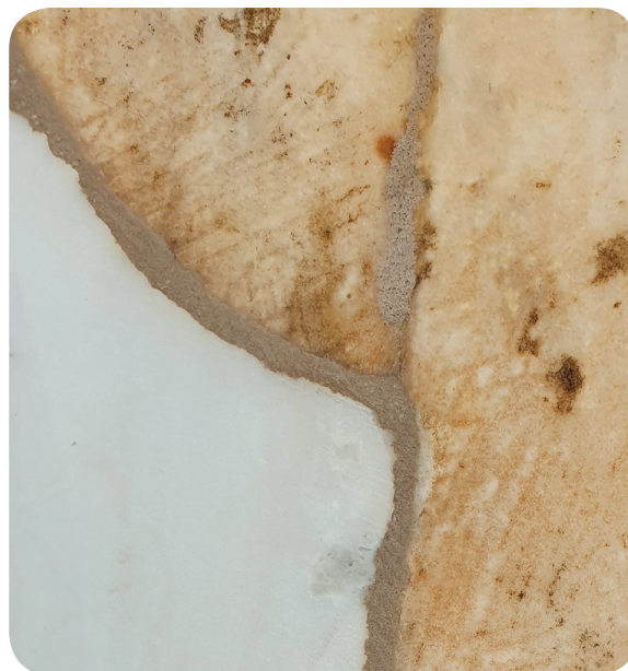
Figure 101: Where the old and new marble pieces touch each other, a layer of mortar is applied: (Barou, n.d.)
