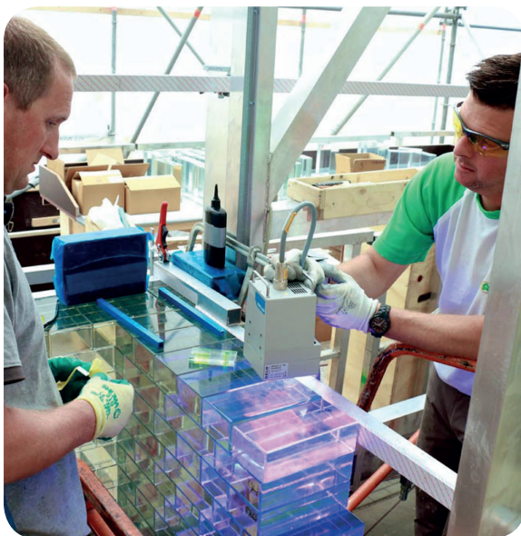
Figure 61: Adhesively bonded glass bricks in the Crystal Houses project, source: (MVRDV, 2016)
