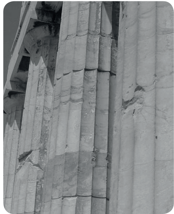
Figure 72: Displacement of drums in the Parthenon columns are often caused by seismic activity, source: (Lambrinou, 2010)
