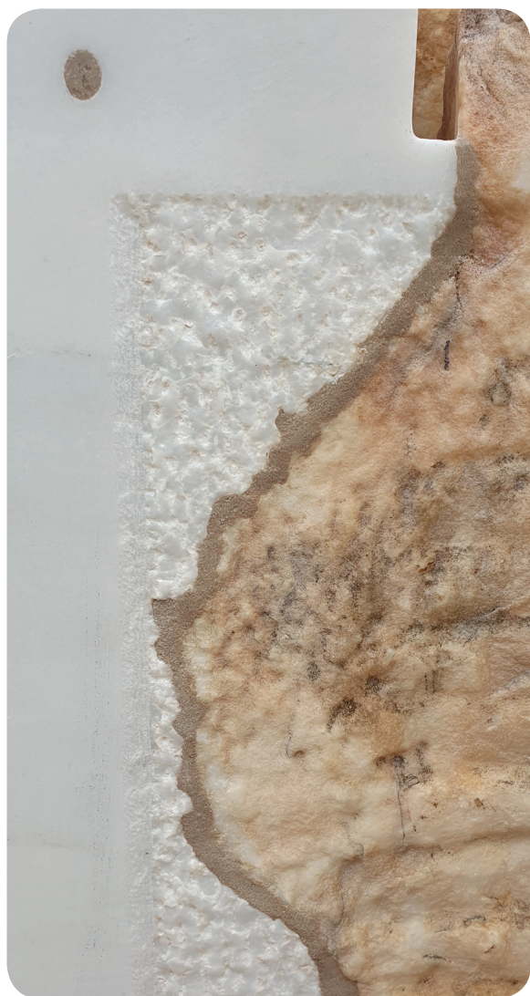
Figure 106: Marble to marble connection filled up with mortar, source: (Barou, n.d.)
