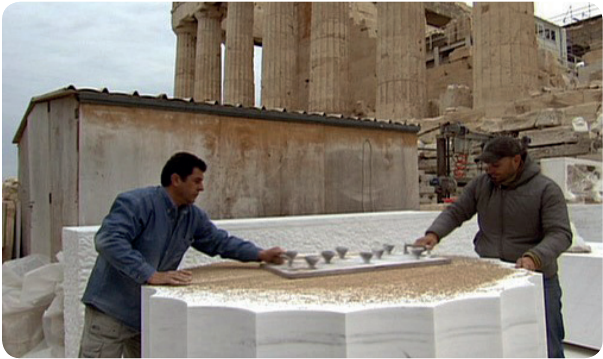
Figure 80: The final sanding process is still done as in ancient times. With this metal plate, which is grinded over the sand, an accuracy of one twentieth of a millimeter can be reached, source: (Glassman, 2008)
