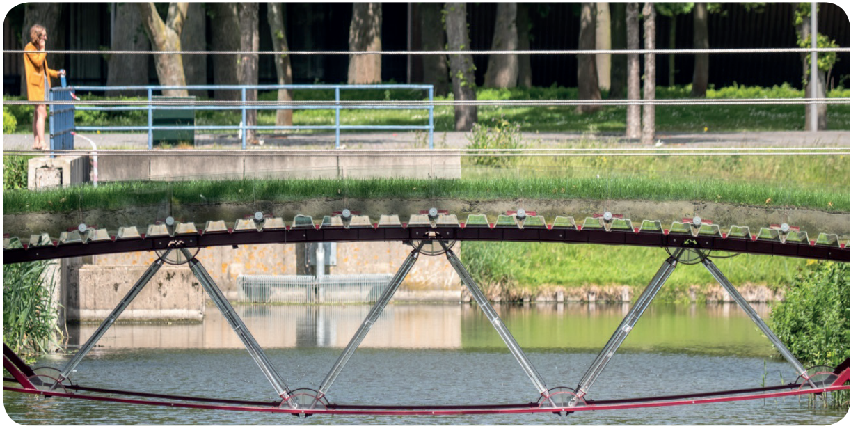
Figure 29: Example of an Extruded Glass structure in the form of a truss bridge, source: (Snijder et al., 2018).
