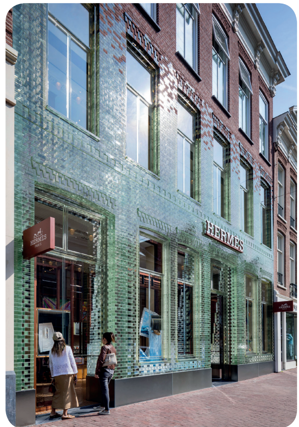
Figure 22 & 23, The soda lime glass blocks from the Crystal Houses are very transparent from a perpendicular view, but looking from an angle, the reflection of the glass becomes more visible, source: (Oikonomopoulou, 2019) top, (MVRDV, 2016) bottom.
