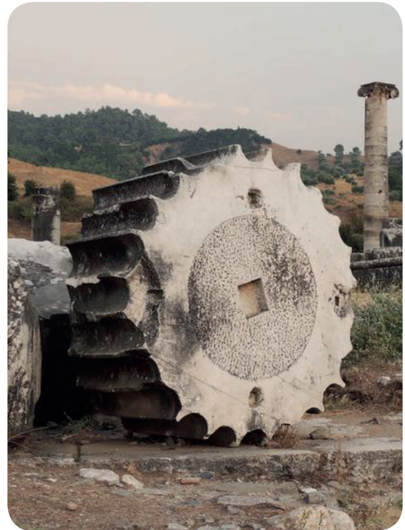
Figure 75: In the middle of this drum in Sardis, Turkey, the carving for the empolion is clearly visible, source: (Cartwright, 2013)
