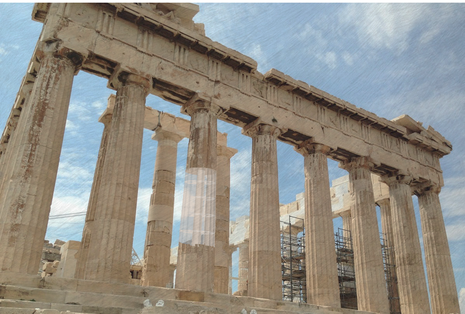
Figure 130: Impression of how a with cast glass restored column, third from the left. The glass is translucent so it is possible to see the marble core within the glass and the interlayers between the drums, edited from: (British Museum, 2012)
