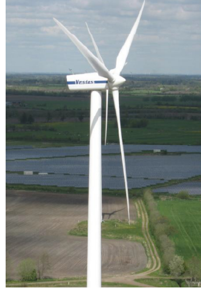
Fig. 3. The Vestas V66 wind turbine under measurement.
