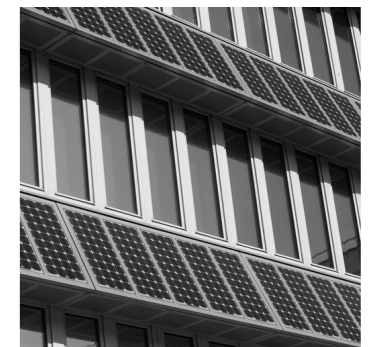
Figure 31 The popularization of wall-mounted solar energy collectors is currently limited by economic costs, the bearing capacity of the supporting wall, and aesthetic considerations.
