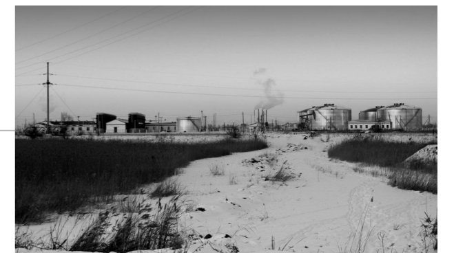
Oil transferring station
