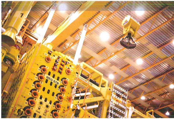
Åsgard modules near completion.
